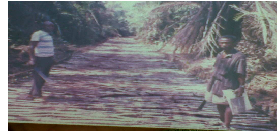
4.Travaux route Nanga (suite)
